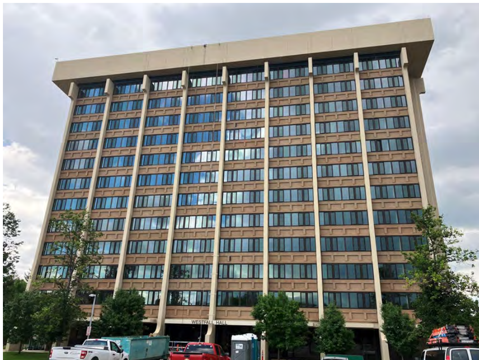
Westfall Hall after Window Replacement
