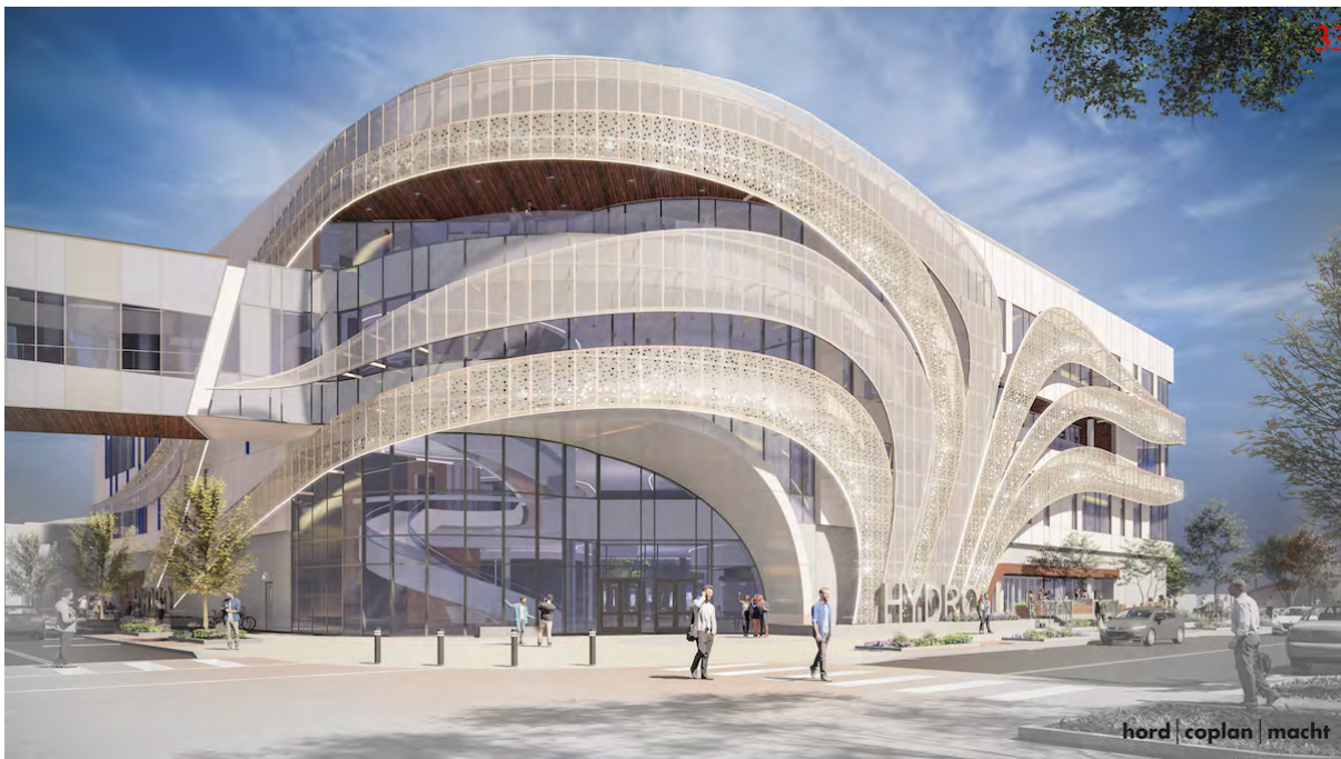
Rendering of the CSU Spur Hydro building, which will open Jan. 6, 2023.
