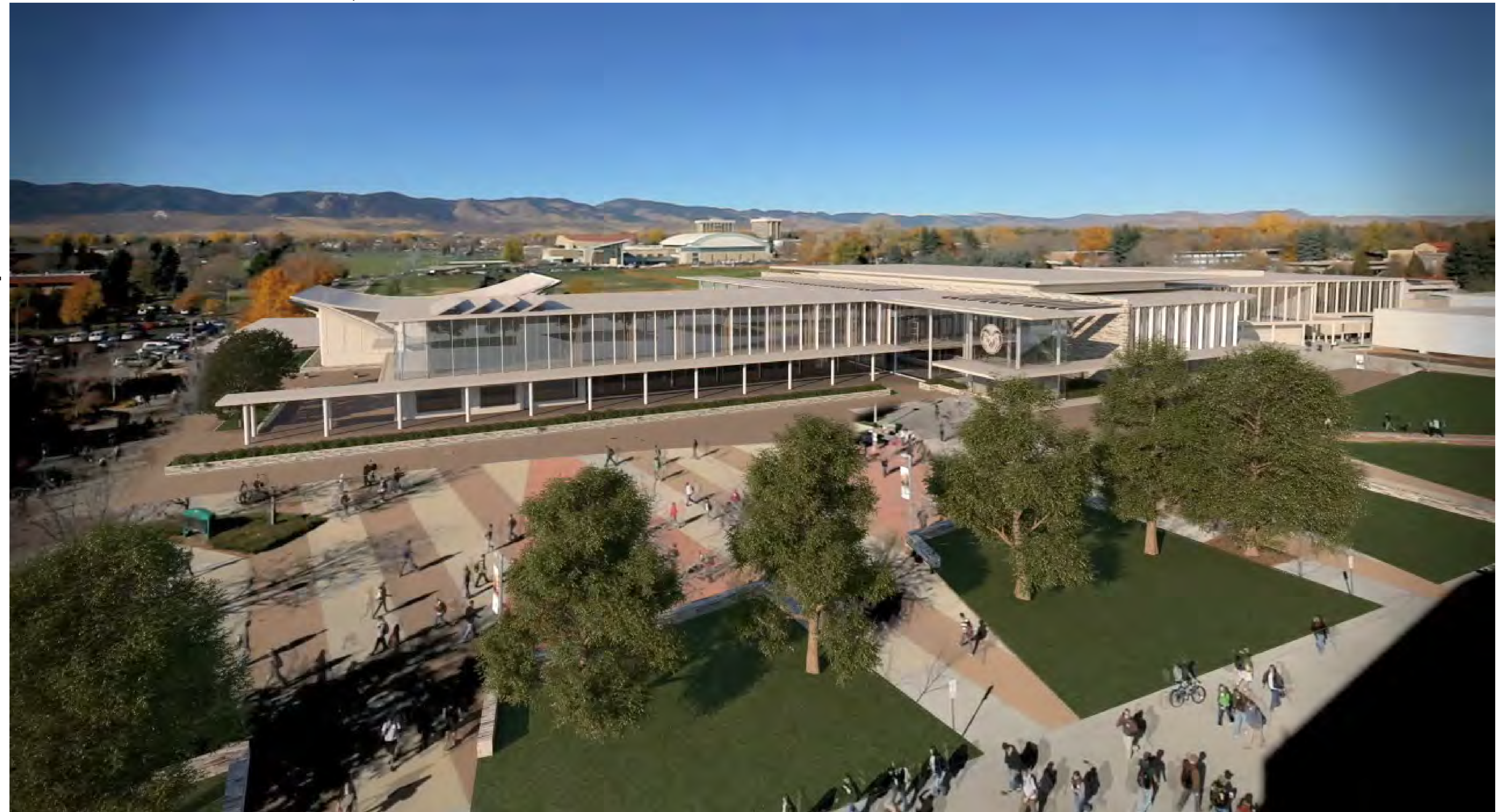
PLAZA FACADE RENOVATIONS AND NEW EAST ENTRY
