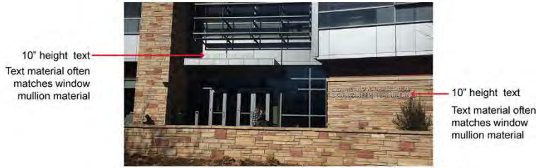
Existing Building Name Sign Mounted on Building
